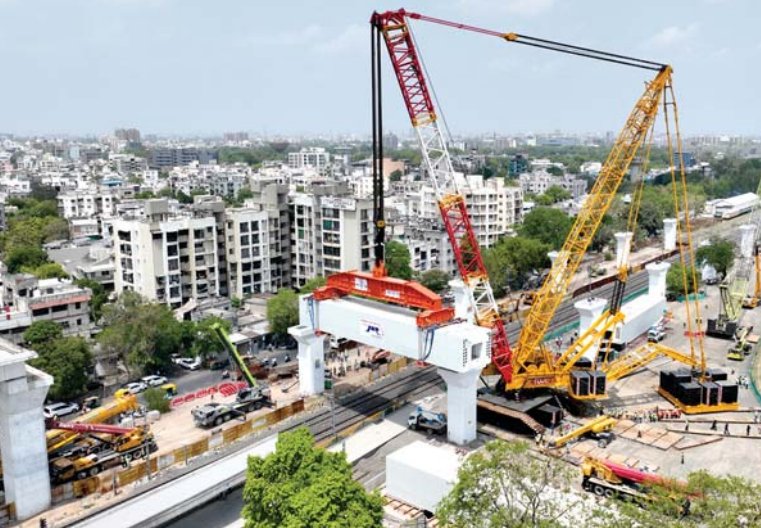
Heaviest portal beam launched over Amdavad-Vadodara rly line in Ahmedabad
